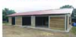
Garage - Abris Chenil
