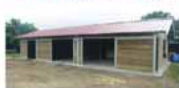
Garage - Abris Chenil
